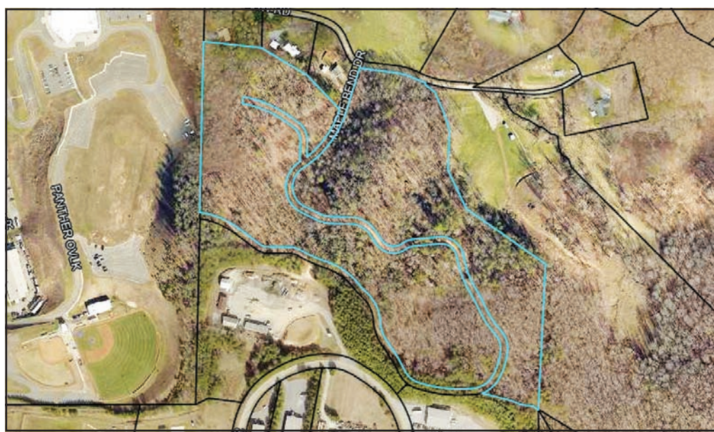
The Union County School System will be acquiring this roughly 32-acre land parcel next to the High School campus to build the new Elementary School. Screenshot/qPublic.net
